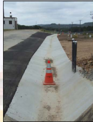
The HDPE injection lines terminate at the northern portion of the trench where they may be connected to the oxidant/activator mixing and conveyance system.
