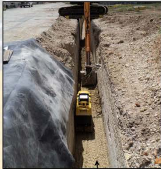
Clay layer added and compacted.
