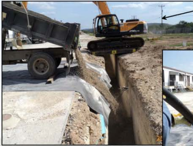
Gravel added and leveled. Injection lines installed.
