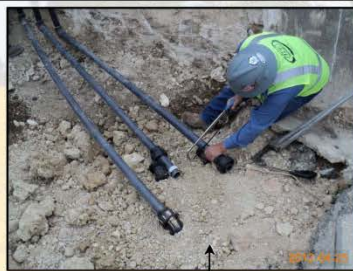
Injection headers installed.
