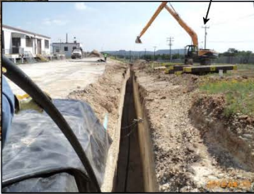
Gravel added and leveled. Injection lines installed.
